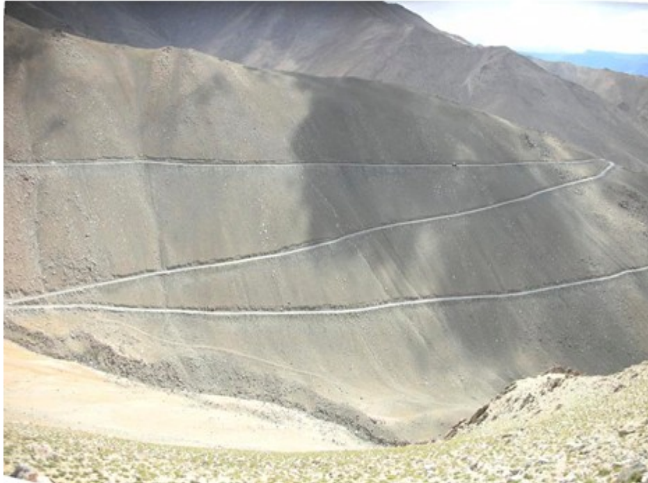
Amazing Zig Zag Roads At Khardung La
